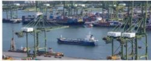
VITAL LINK. Indian trade uses the Singapore port as a major transshipment hub S.L.O.C.H.INDIA
